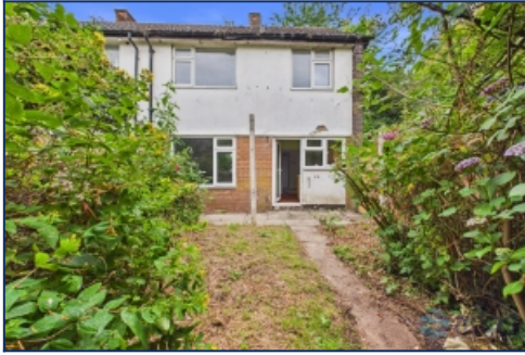
Rear Elevation Of Property
