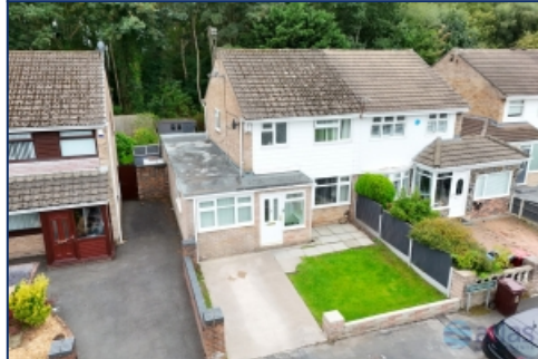
Front Aerial Elevation
