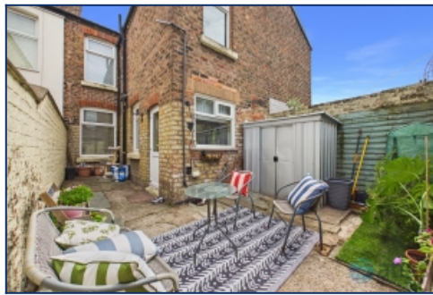
Rear Elevation & Rear Yard
