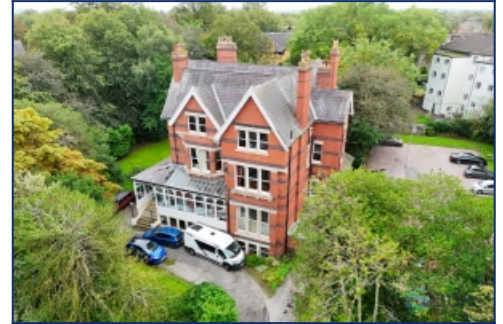
Front Aerial Elevation
