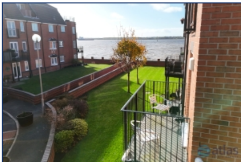
Aerial View Of Balcony
