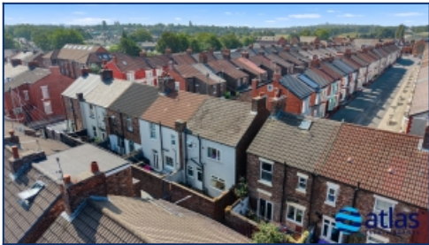
Aerial Rear Elevation
