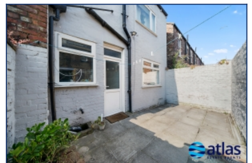
Rear Elevation & Rear Yard
