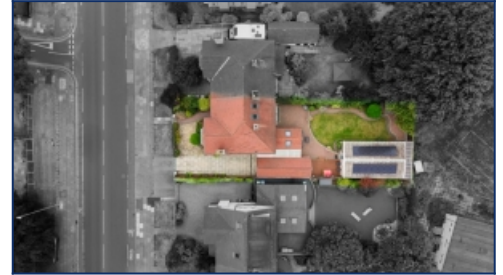
Aerial View Boundary
