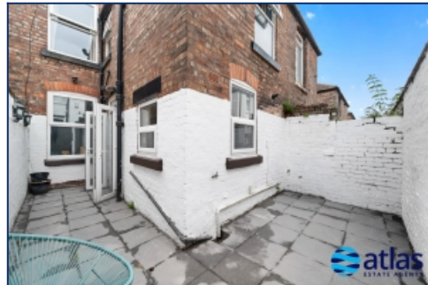
Rear Elevation & Rear Yard
