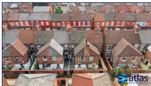
Aerial View Rear Elevation
