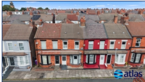
Aerial Front Elevation
