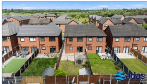
Aerial Rear Elevation
