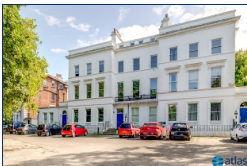
Rear Elevation Of Building
