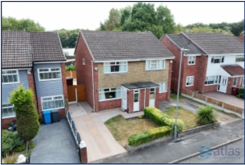
Aerial Front Elevation
