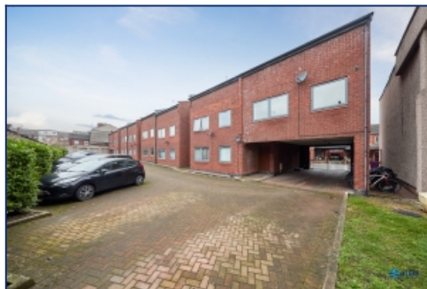
Gated Car Park
