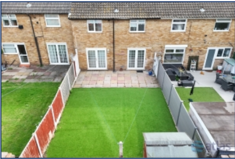
Aerial Rear Elevation & Garden
