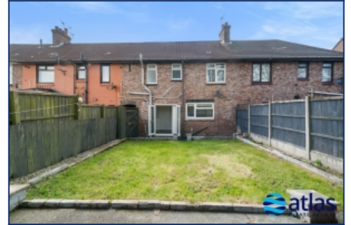
Rear Elevation Of Property
