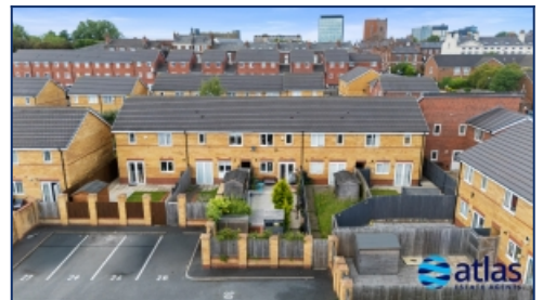
Rear Elevation Of Property
