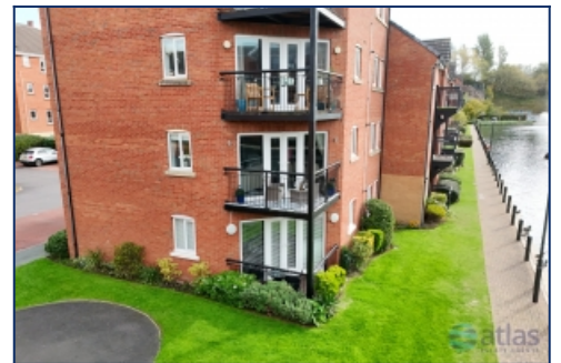
Aerial View Balcony
