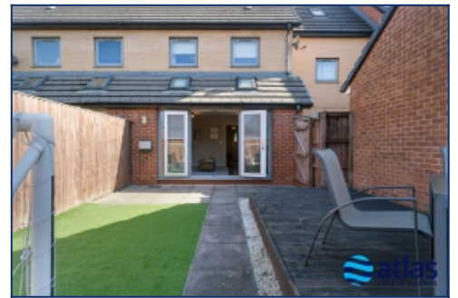
Rear Elevation Of Property
