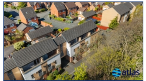
Aerial Front Elevation
