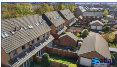
Aerial View Rear
