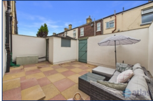
Rear Elevation & Rear Yard
