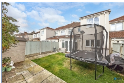
Rear Elevation Of Property
