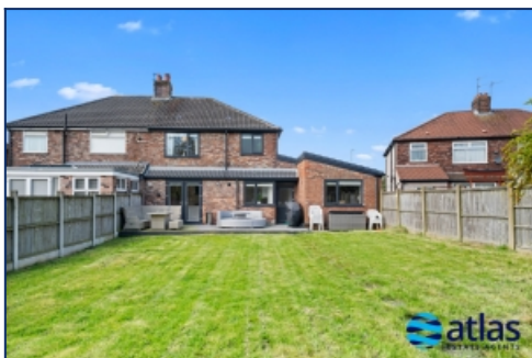
Rear Elevation Of Property
