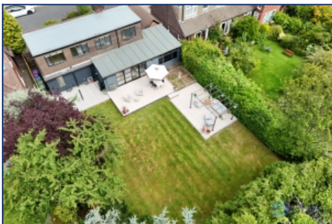
Aerial Rear Elevation & Garden
