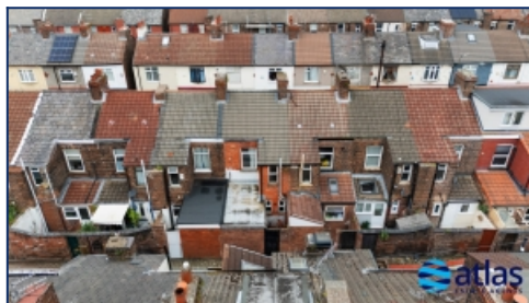
Rear Elevation Of Property
