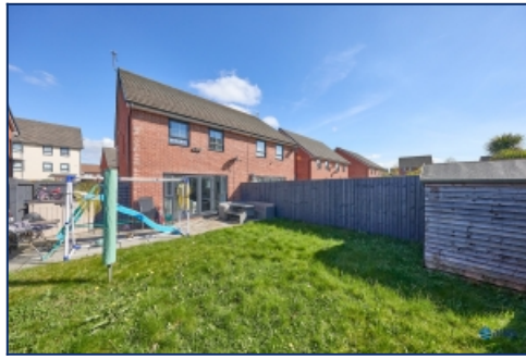
Rear Elevation Of Property
