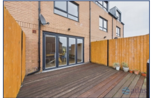
Rear Elevation Of Property
