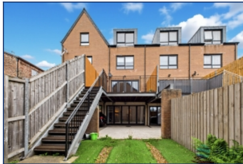
Rear Elevation Of Property
