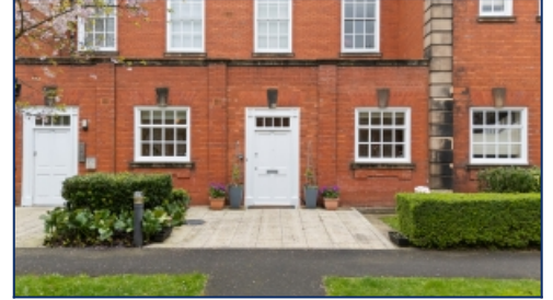
Front Elevation Of Property
