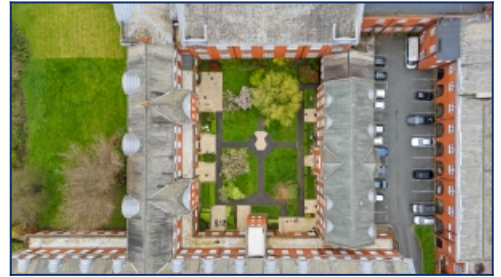
Aerial View Of Building
