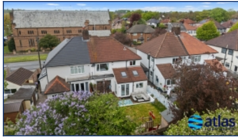
Aerial View Rear
