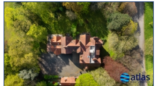
Aerial View Of Building
