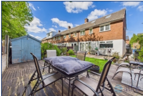
Rear Elevation Of Property
