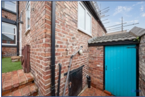
Rear Elevation Of Property
