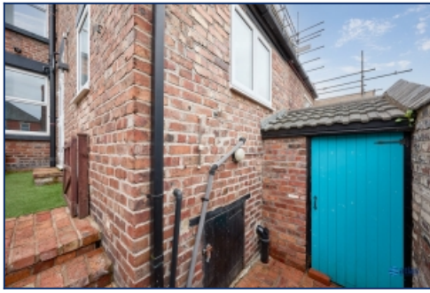
Rear Elevation Of Property
