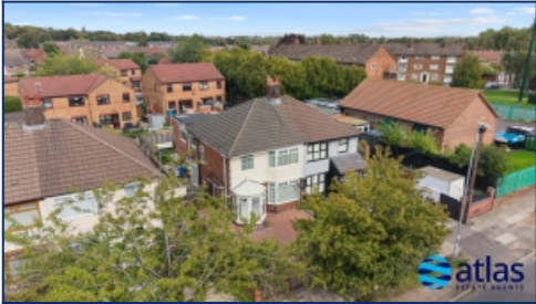
Aerial Front Elevation
