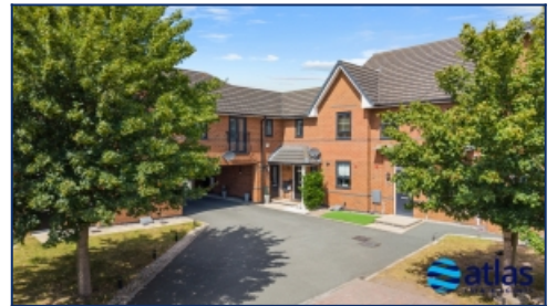
Aerial Front Elevation
