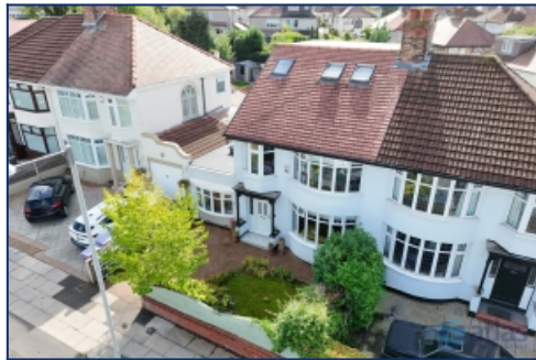
Aerial Front Elevation
