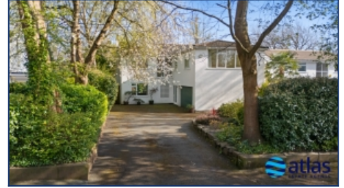
Front Elevation Of Property & Driveway
