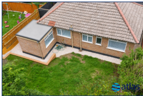
Aerial Rear Elevation & Garden
