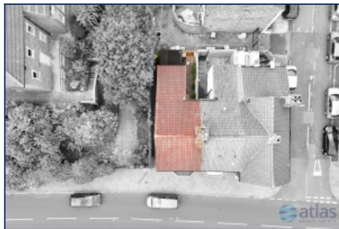
Aerial View Boundary
