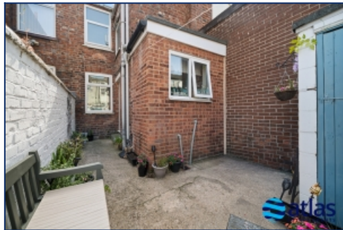
Rear Elevation & Rear Yard
