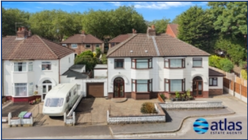
Aerial Front Elevation
