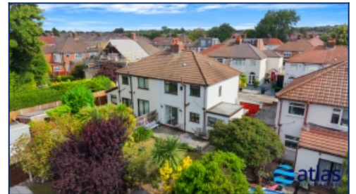
Aerial Rear Elevation
