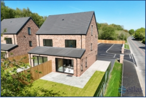
Aerial Rear Elevation
