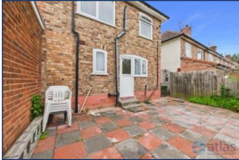
Rear Elevation Of Property
