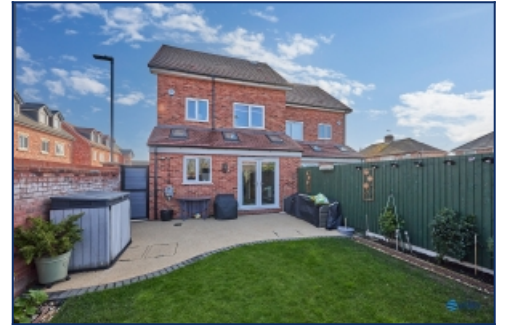
Rear Elevation Of Property
