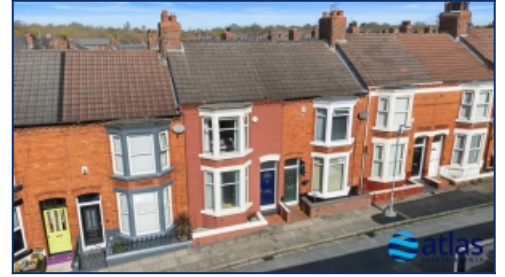
Aerial Front Elevation
