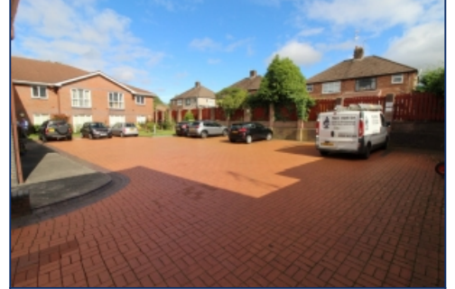
Communal Car Park
