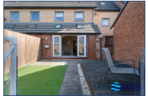
Rear Elevation Of Property
