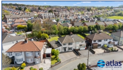
Aerial Front Elevation
